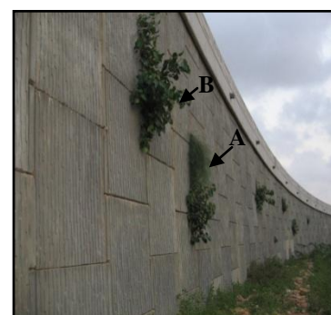
Fig.15. Group of ediphytes growing from the ramp crevices of newly constructed Lyari Express Way Ramp A-B = refer to Fig.14.
